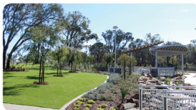
Considered - Planted drainage retention
