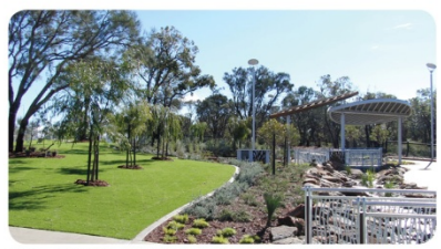
Considered - Planted drainage retention
