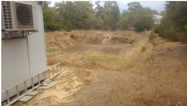
Council clearance of drainage pit within Duncraig compound.
