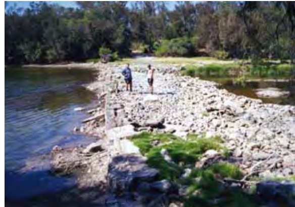
Weir at the downstream end of Glen Avon Pool (Photo courtesy Bernard Kelly)
