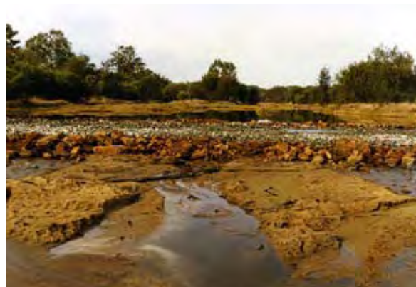
Riffle constructed upstream of Burlong Pool to trap sediment (Photo courtesy Bernard Kelly)
