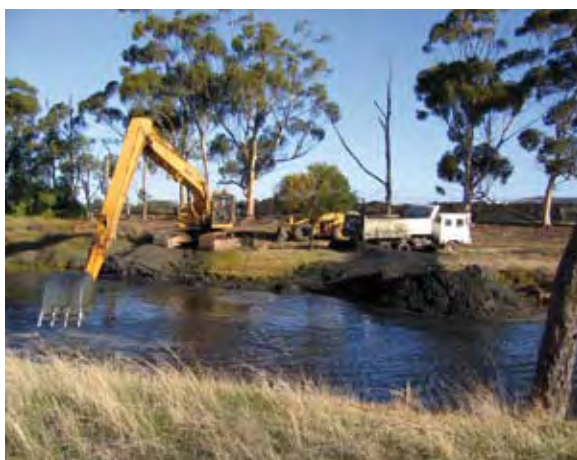
Long-reach excavator removing sediment from the pool. (Photo courtesy Michael Allen)
