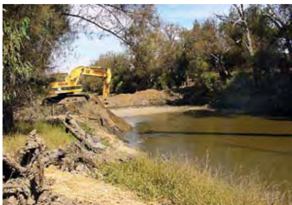
Excavation of Railway Pool in 2002 (Photo courtesy Nina King)
