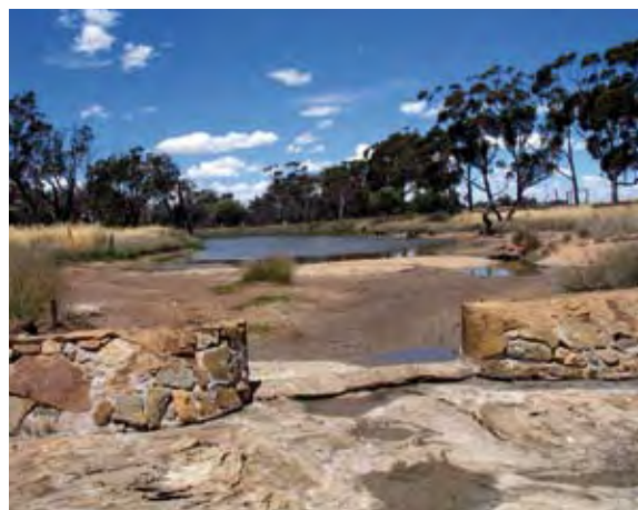
Weir-like structure at the downstream end of One Mile Pool. (Photo courtesy Prue Dufty)
