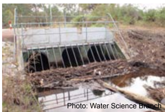
A gross pollutant trap covered in wood and other debris following heavy rainfall, June 2011.
