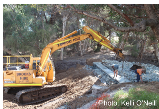
Constructing a rock riffle on Bannister Creek, April 2012.
