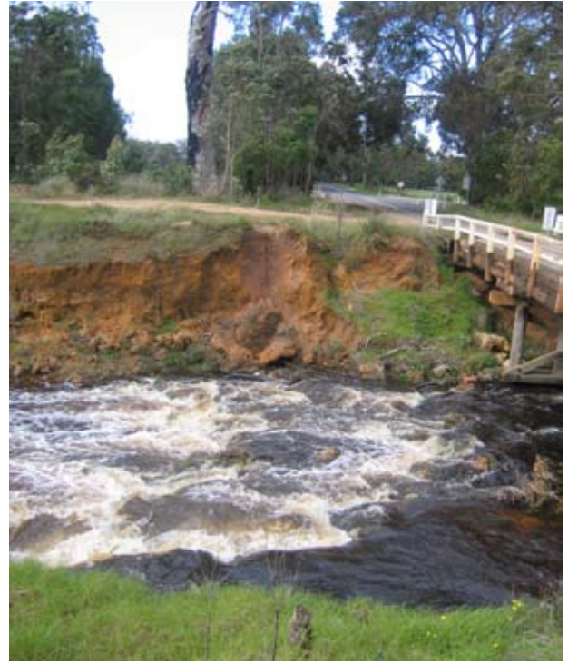
Photo 10 D2 grade foreshore
