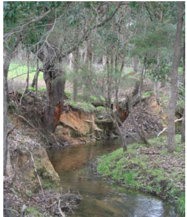
Photo 8 C3 grade foreshore
