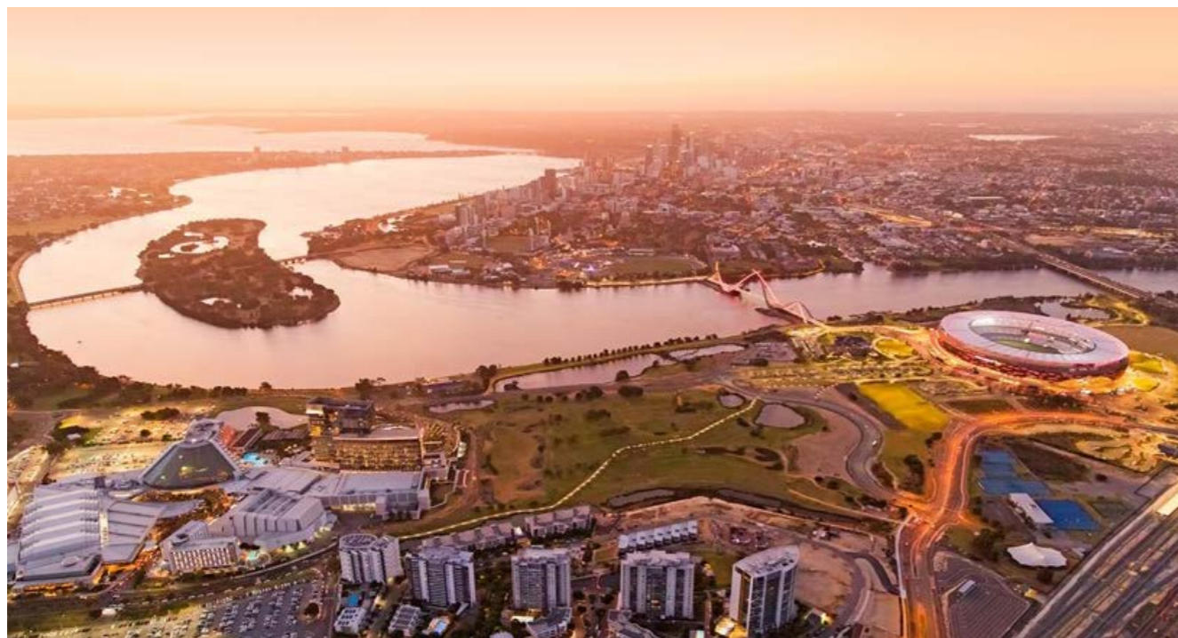
Aerial view of Structure Plan Area looking towards Perth CBD.
