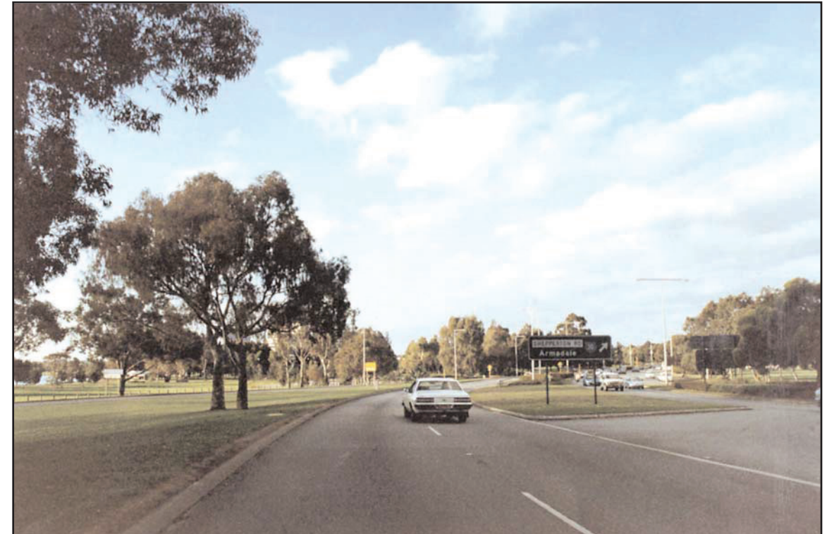
View 8 - Approaching Great Eastern Highway
