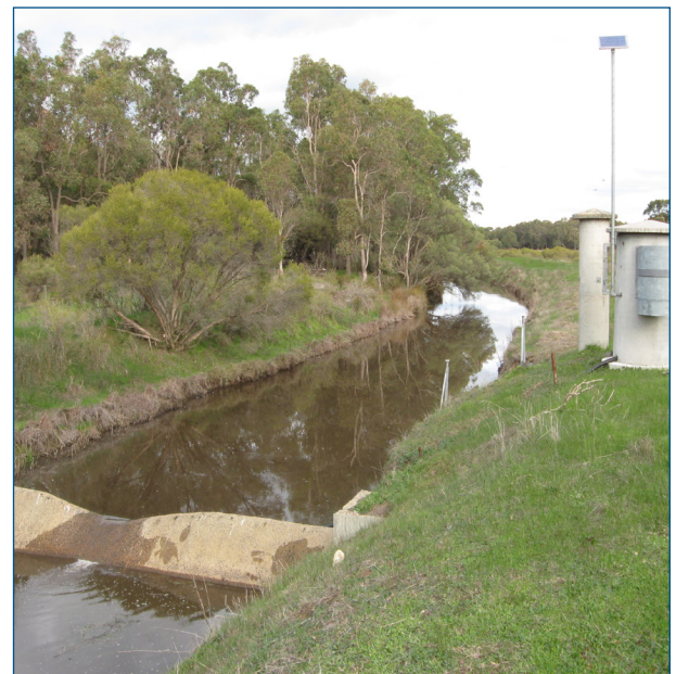
Coolup South Main Drain 613027 – May 2005
