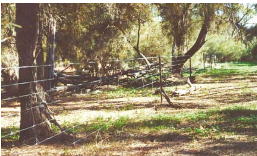
Fence condition: GOOD
