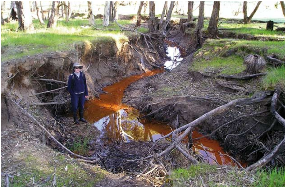
Photo 7 Deep gully erosion in section JB006
