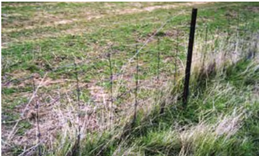
Fence in moderate condition
