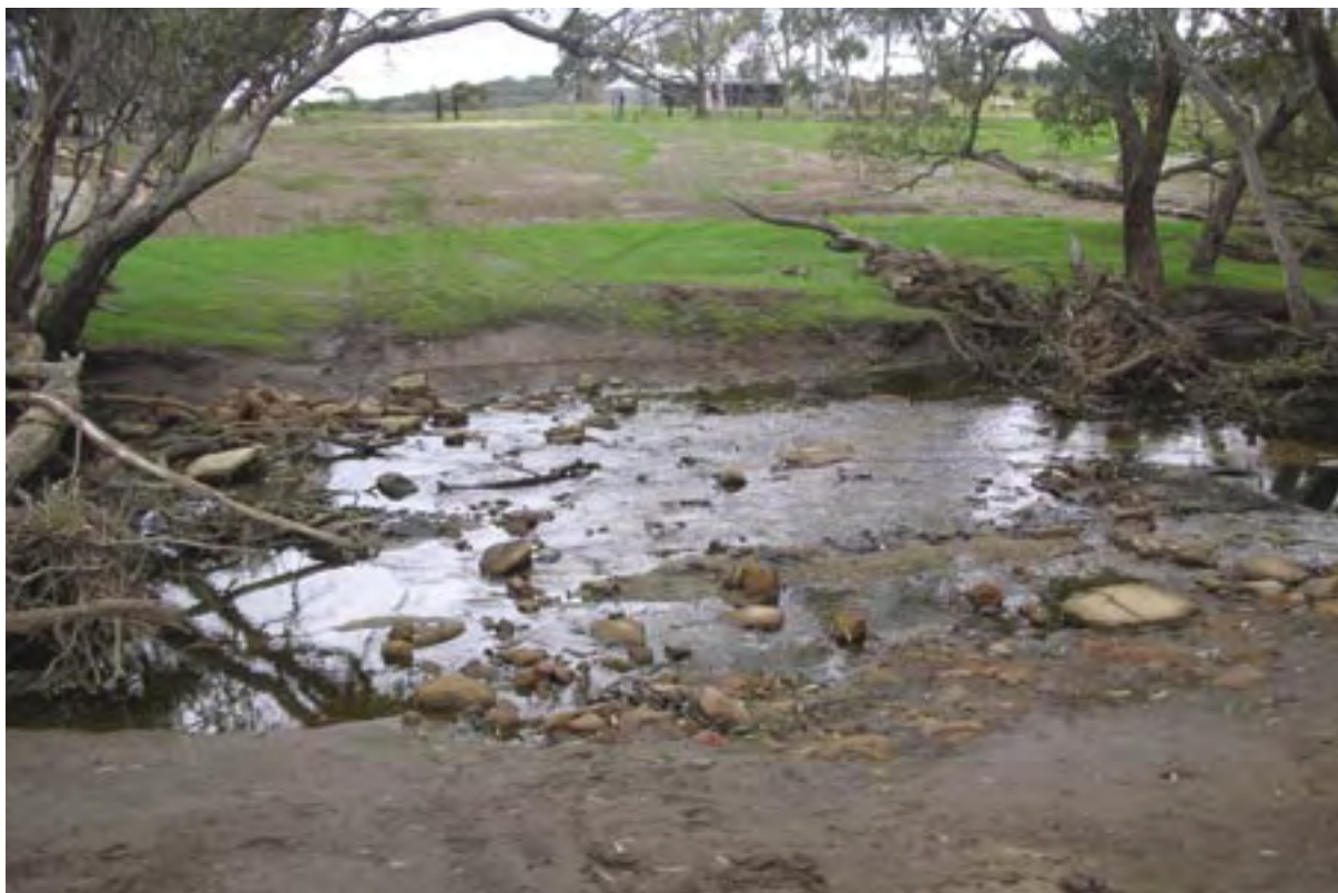
Photo 6 Farm crossing stabilised with field stone
