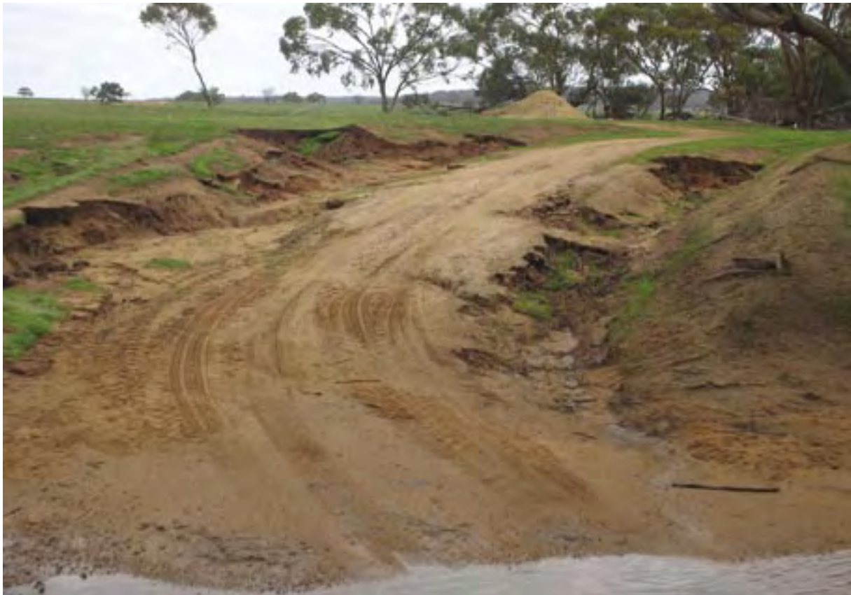
Photo 9 Erosion and washout of a track crossing the Dale River South
