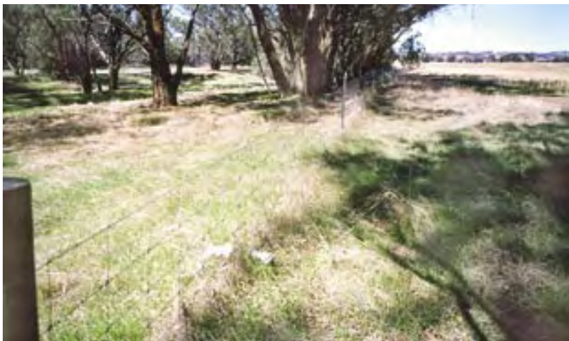
Fence in good condition
