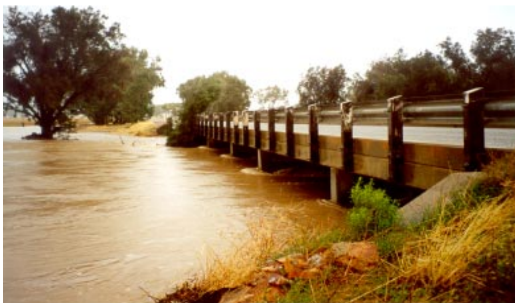
The Mackie River in flood during January 2000 at the bridge over the York-Quairading Road in York. [Photo by Daniel Ryan]
