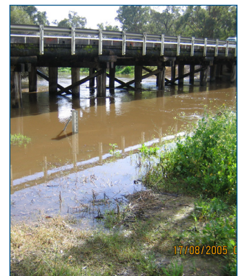
Clifton Park at the Old Bunbury Road Bridge – August 2005
