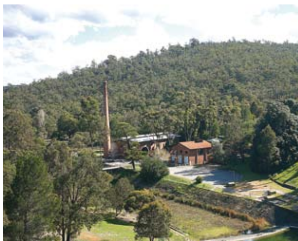
2 Pumping station beside Helena River from Weir (IMG_0003)
