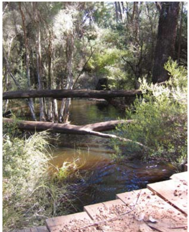
38 Darkin River at Nockine Road Bridge (Darkin River Nockine Rd crossing-2)
