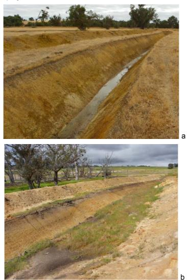
Figure 8 Soil profiles of the drain showing varying depths of sand over clay soil at (a) Transect 1 and (b) Transect 4
