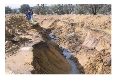
Figure 7 Drain slumping
