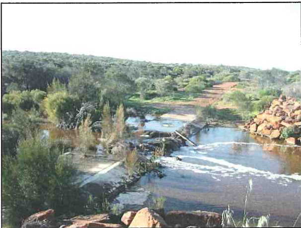
Photograph 3: The old Port Gregory Road crossing although slowly eroding away is still obstructing small to medium flows
