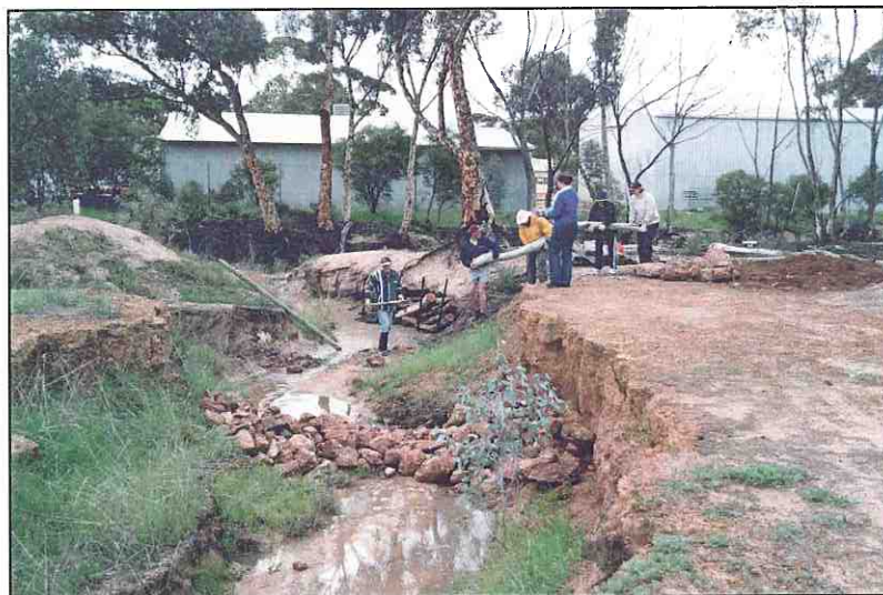
Photograph 13: Rock riffle structures and logs placed instream can arrest erosion and get a river on the road to recovery.
