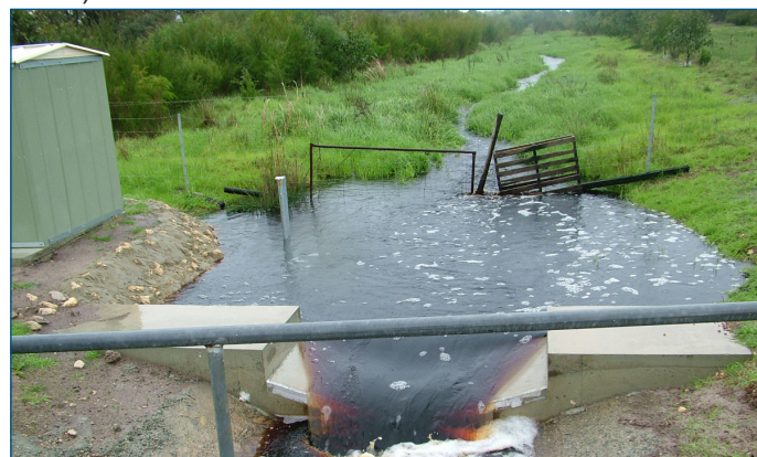
Upstream view of Gull Road Drain – June 2005
