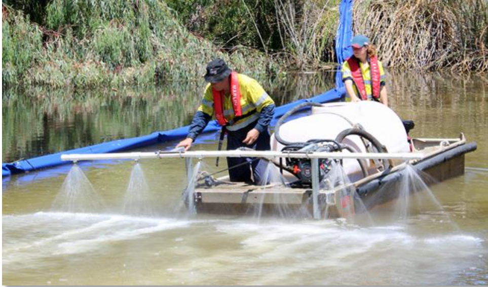
Figure 6: Clay application from a moving barge equipped with a petrol pump and spray boom.
