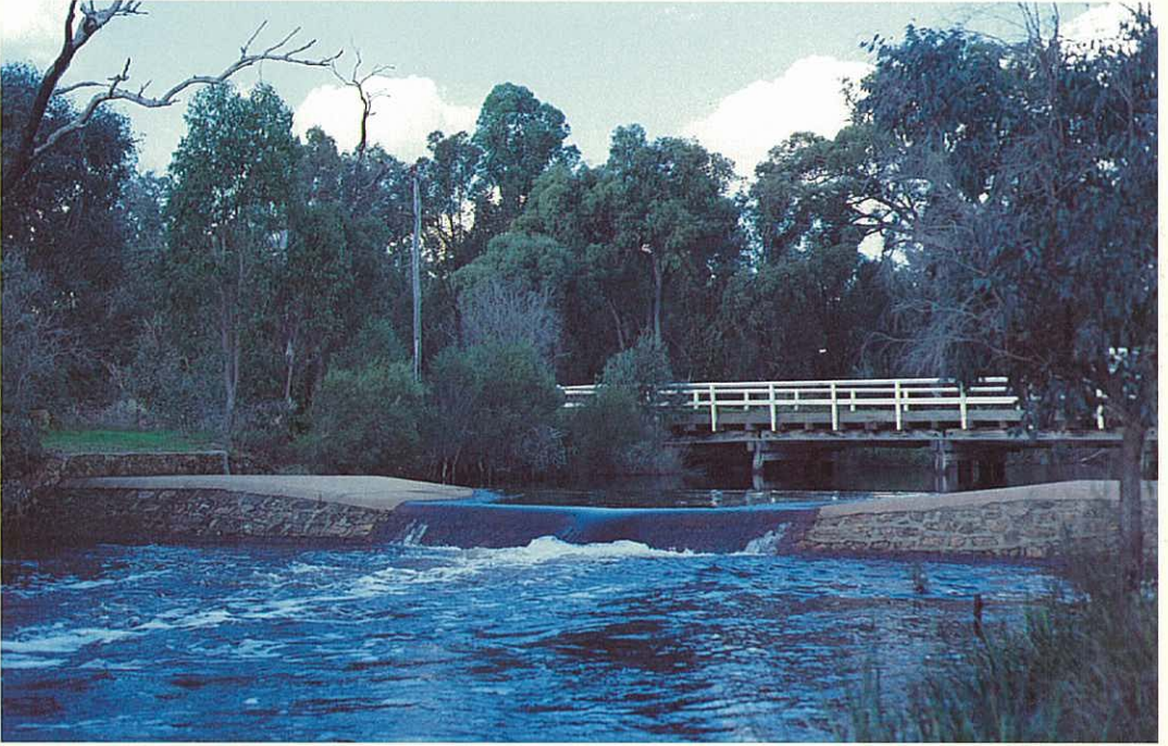
EVERY WINTER AND SPRING THOUSANDS OF NATIVE FISH, ATTEMPTING TO MOVE UPSTREAM, GATHER BELOW THIS WEIR AND OTHERS LIKE IT THROUGHOUT THE SOUTH-WEST. OCCASIONALLY WEIRS LIKE THIS FLOOD-OUT AND THE FISH CAN MOVE UPSTREAM. LARGE DAMS, CULVERTS AND FENCES JAMMED WITH DEBRIS ALSO BLOCK FISH MOVEMENT. PHOTO: L.PEN
