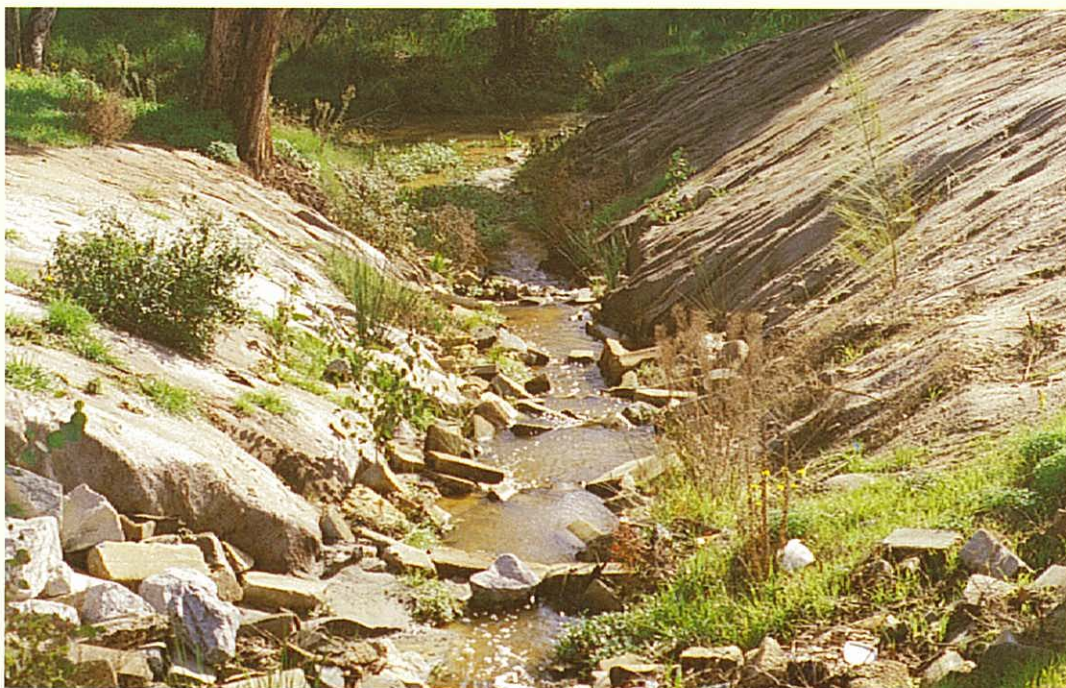
ROCKS AND BROKEN CONCRETE ARRANGED AT THE BASE OF THE SOUTHERN WOOD CREEK (CITY OF GOSNELLS IN PERTH) TO ARREST HEADCUTTING AND CREATE A CASCADE EFFECT. MESH HAS ALSO BEEN ARRANGED ON THE BANKS PRIOR TO REVEGETATION. PHOTO: L. PEN
