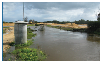
During diversion – 10 July 2007
