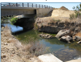
Before bank stabilisation – March 2009
