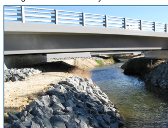
After bank stabilisation – June 2009
