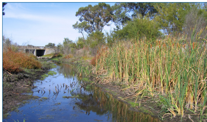
Meredith Drain, downstream of Johnston Road, looking upstream to the gauging station – March 2009
