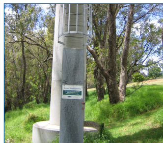
View of the gauging station at Pinjarra – December 2005
