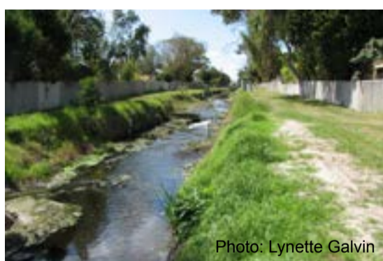
Mills St Main Drain.
