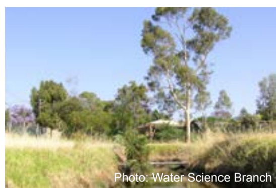
Mills St Main Drain.
