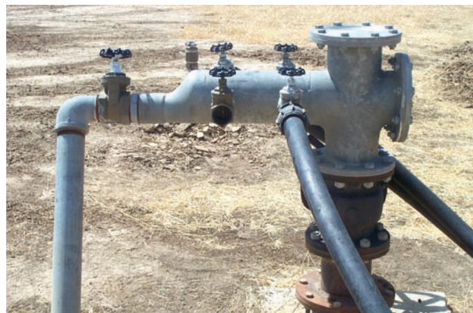
Water supply under control
