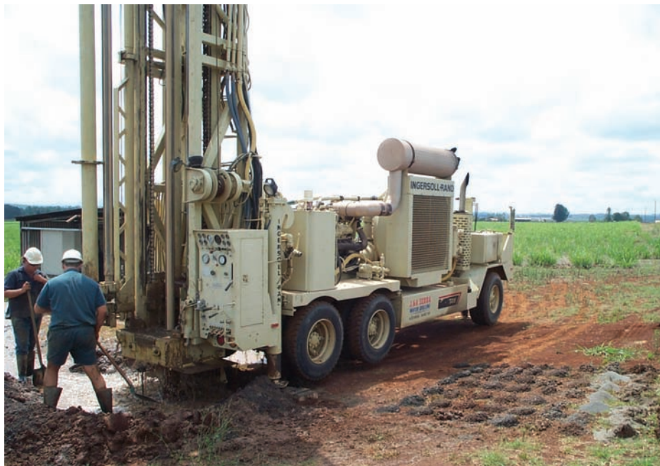
Laying out samples of drill cuttings
