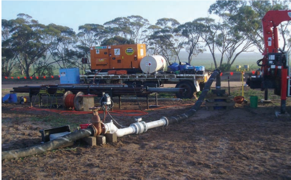
Bore yield testing
