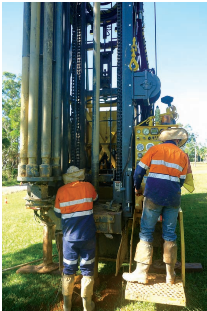
Rotary air drilling
