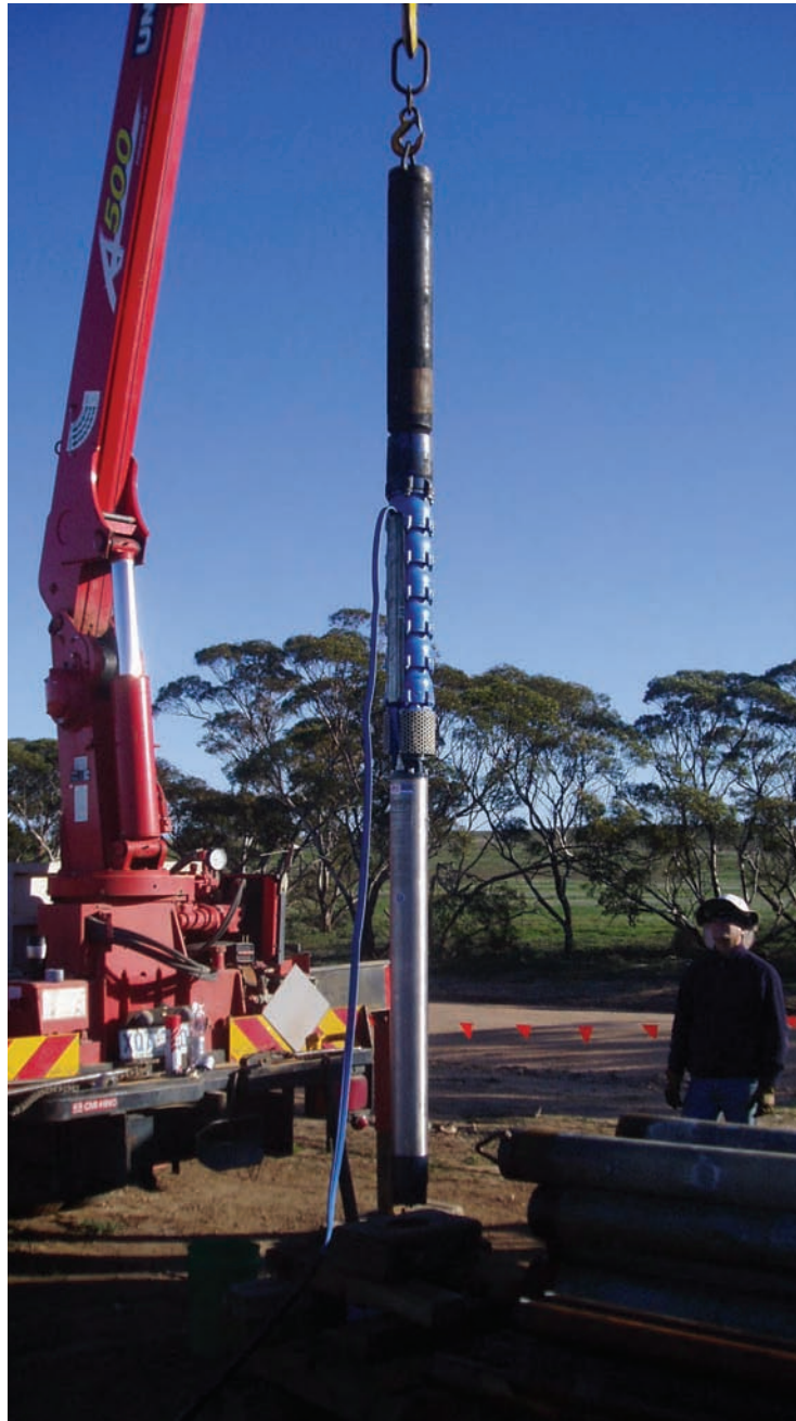
Submersible pump being lowered into a bore
