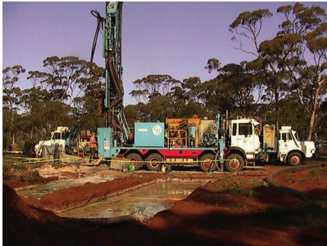
Rotary mud drilling
