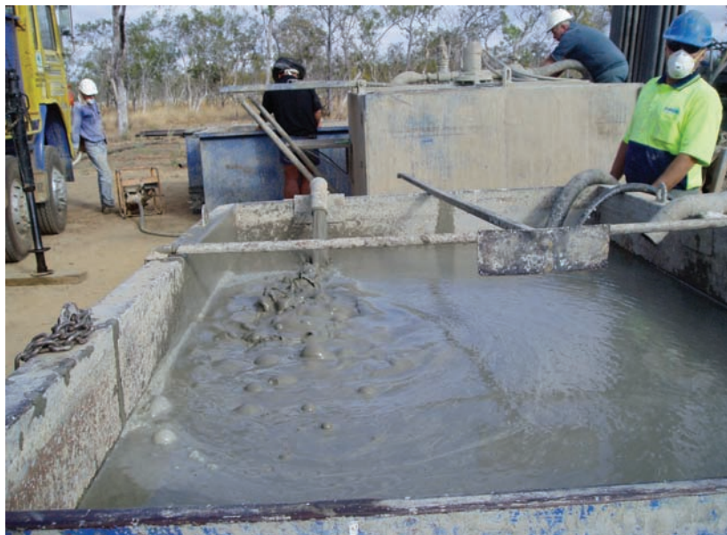
Cementing the bore
