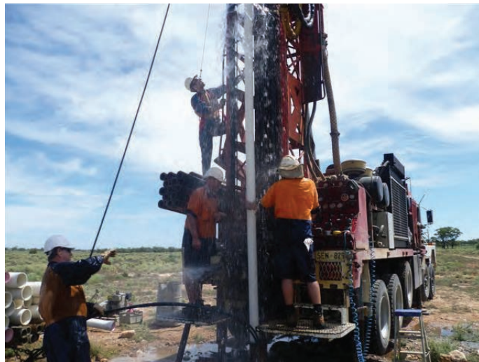
Running casing into the hole Photo courtesy of Kangarilla Drilling Pty Ltd.
