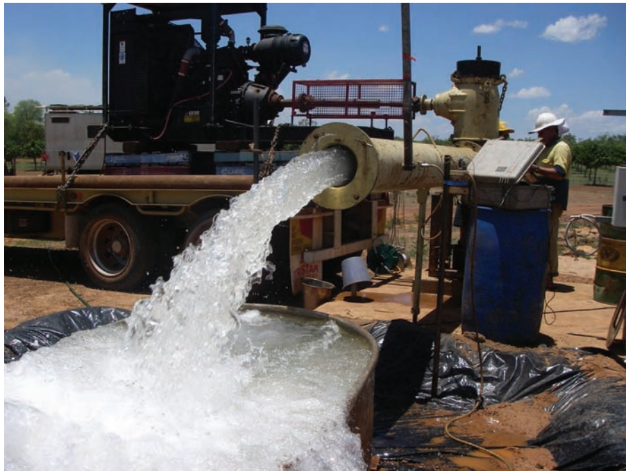
Test pumping an irrigation bore
