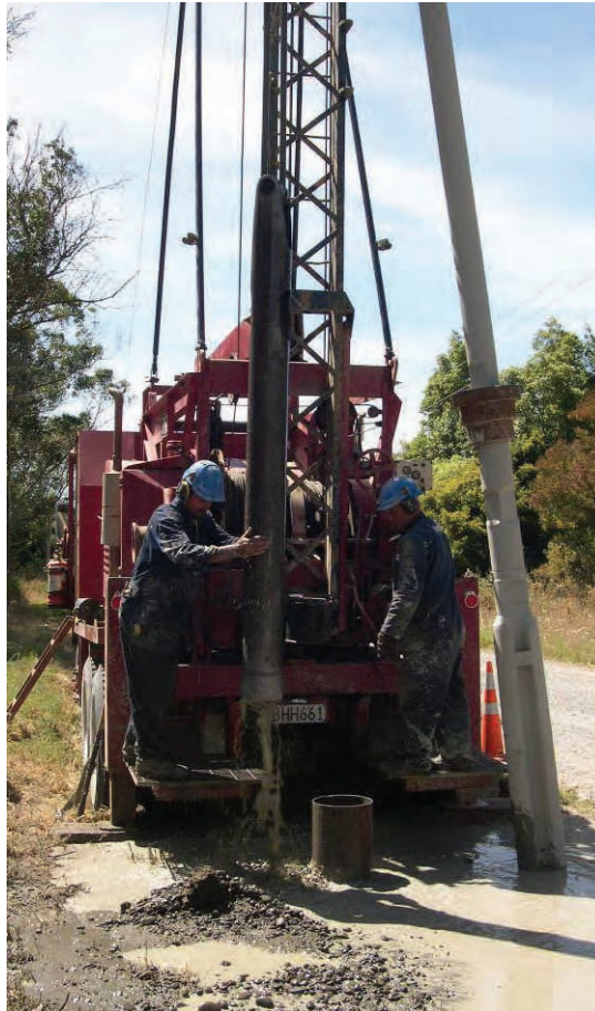
Cable tool drilling
