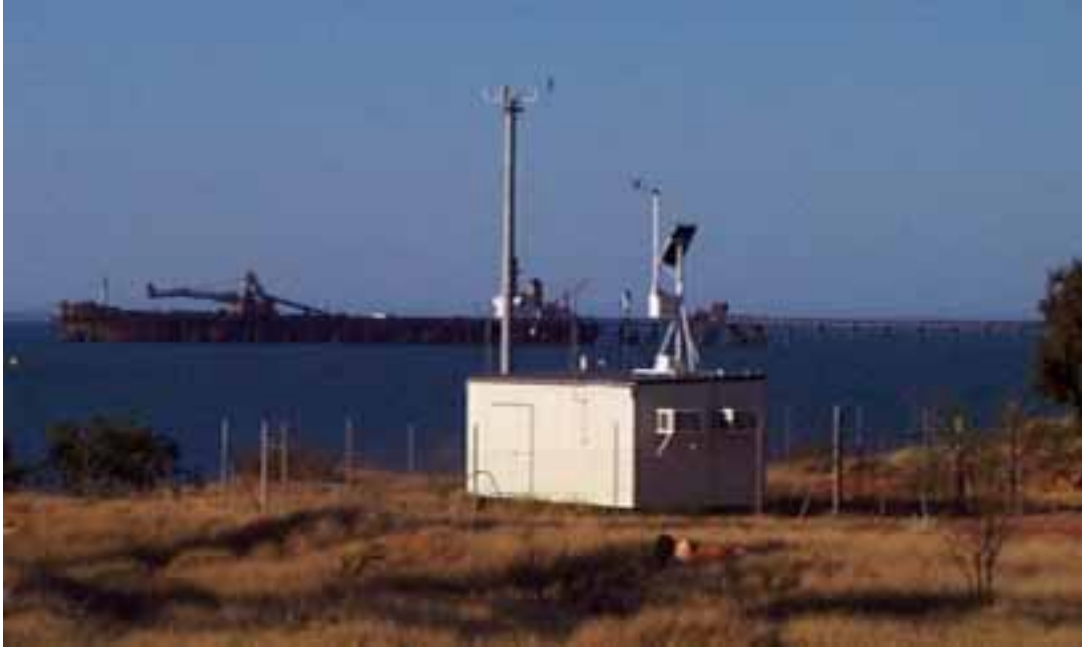
Figure 3.1 Dampier AQMS - looking north, with Parker Point jetty in background.
