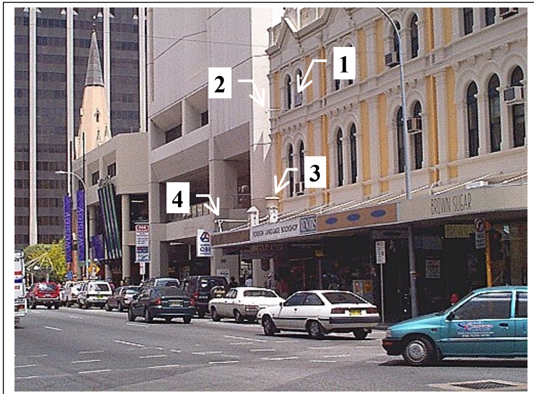
Figure 4.2. External aspect of the Queens Building Performance Monitoring Station: 1 is the actual monitoring room, 2 is the nephelometer inlet, 3 is the PM 10 sampler and 4 is the inlet sample tube.
