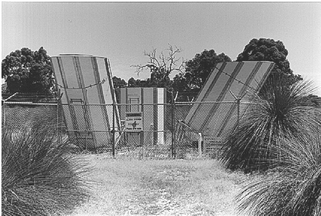
Figure 7.2 - Sodar Compound located at Cullacabardee.
