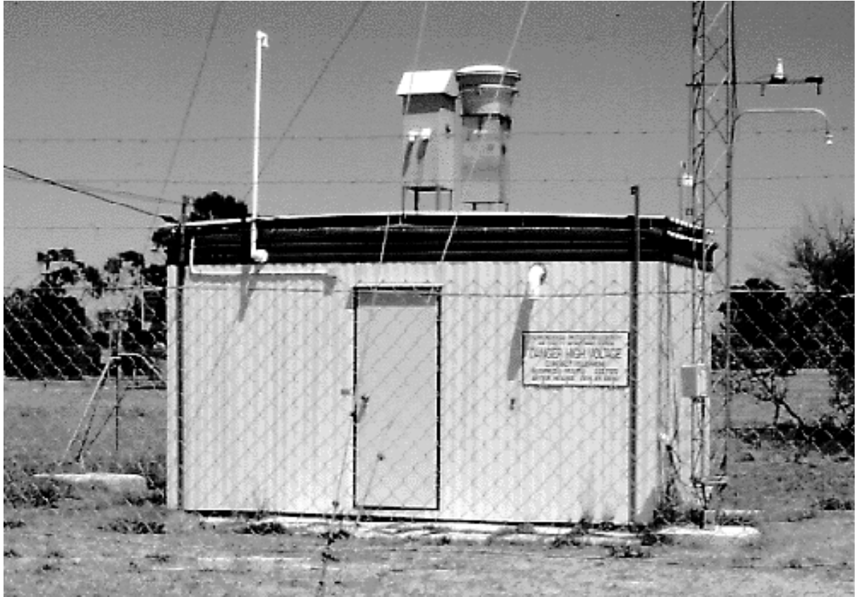
Figure 3.1 - Air quality monitoring shed at Caversham.
