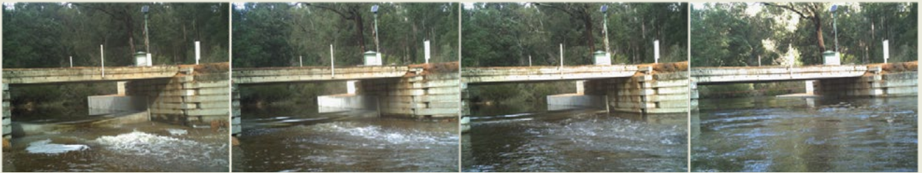
Figure 14 Detailed assessment of water levels and flow to determine requirements to support fish passage (Yanmah Brook, Western Australia).
