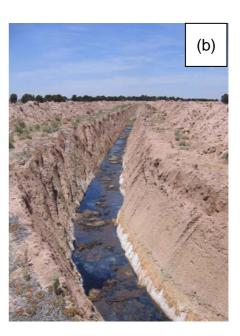
Figure 23 In-drain composting bed (a) after construction and (b) 6 months operation (during Trial period 2)
