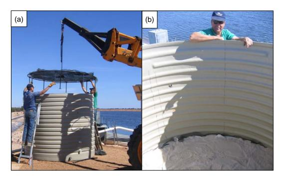
Figure 41 Construction of the percolation tank reactor illustrating (a) lowering the percolation tables through the top of the tank and (b) placing lime-sand on fine nylon mesh on each table
