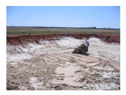
Figure 27 Levelling the lime-sand bed in the floor of the pilot evaporation basin
