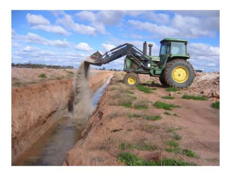
Figure 13 Loading lime-sand into a drain using a front-end loader: note the opening of the levee banks to allow access
