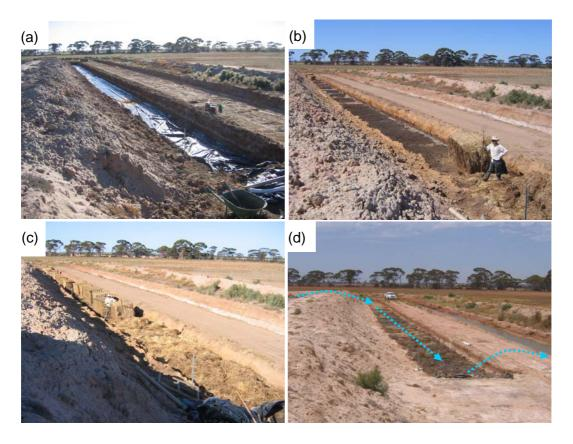
Figure 35 Composting wetland cell construction stages: (a) empty pit (b) after loading sheep manure (c) loading straw bales and (d) after filling with water. The blue arrows indicate the flow path of the water through the wetland from the evaporation basin to sump drain.
