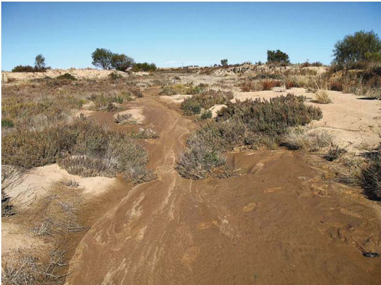
Photo 8 Erosion and sedimentation problems in a reach of Mooranoppin Creek (Photo: S. Mehmet)
