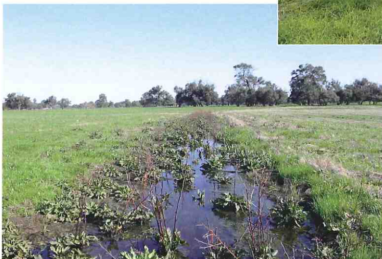
D3 grade foreshore. This drain is approximately 1 metre wide, with very low flows. Due to the low flows, the grasses and clovers are able to hold the bank together and there is little erosion occurring,
