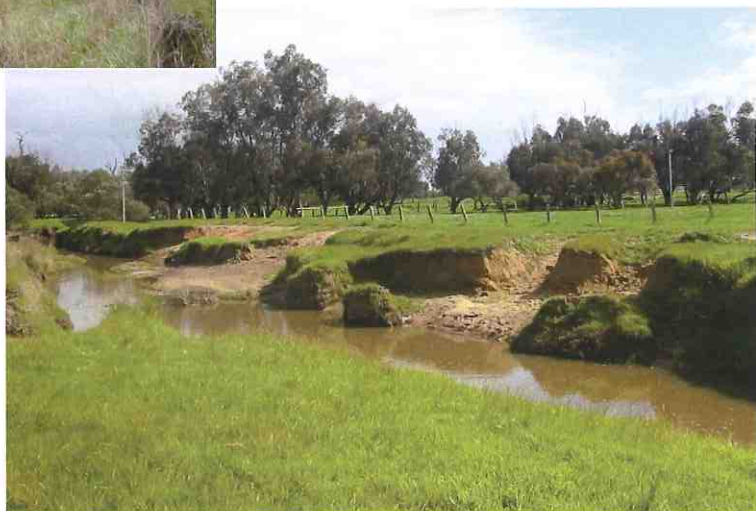
D2 Grade foreshore. No fringing vegetation remains and banks are freely eroding, resulting in massive sediment transport downstream, loss of productive land and serious downstream water quality issues.
