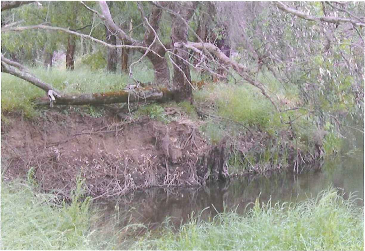
C3 Foreshore. Note the extensive bank erosion and the understorey consists entirely of annual weeds.
