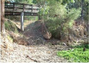
PP69: Bank damage as a result of storm water entry
