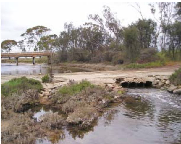
Photo 30: Culvert and Bridge at the Brookton-Kweda Road crossing in Photo Section 18
