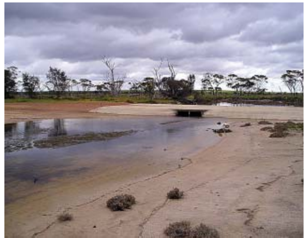
Photo 32: Substantial farm access crossing in Photo Section 18
