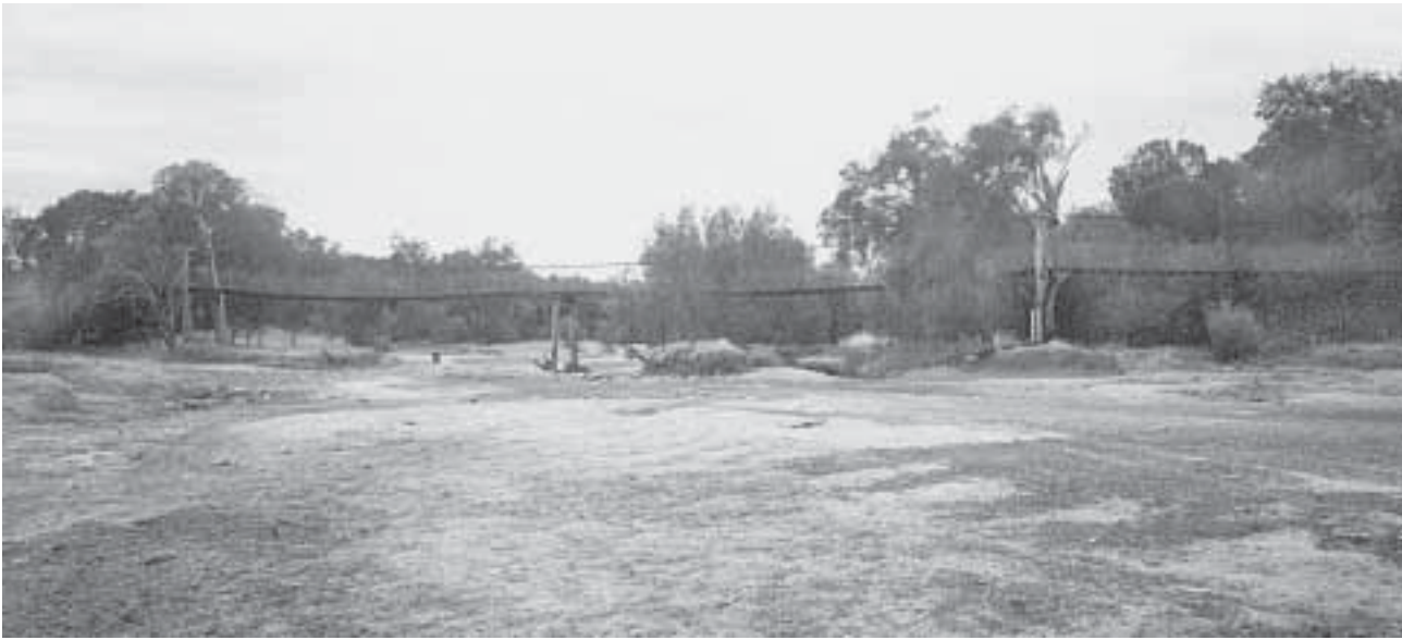
Photo 17: The Swinging Bridge at Muresk
