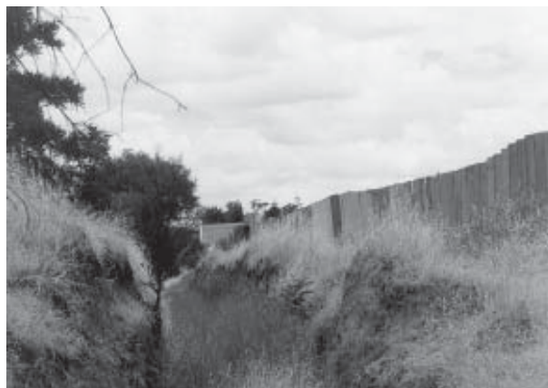
Stormwater drain, Northam. [Photograph courtesy of C Ryan]
