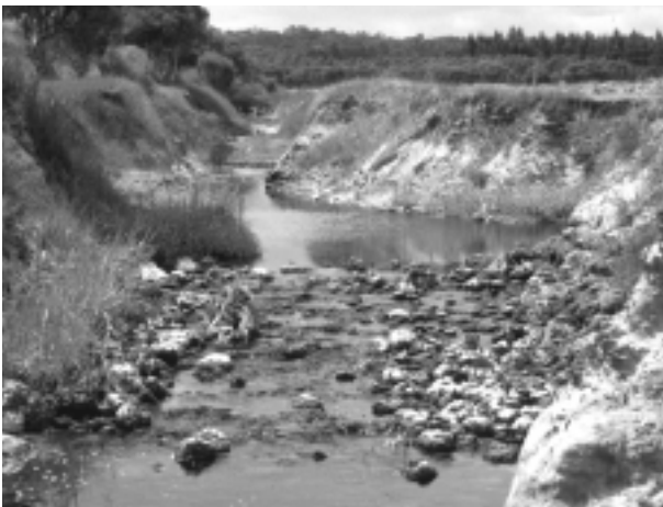
Figure 8. An artificial riffle constructed in a straightened section of a creek is intended to slightly slow water and sediment movement, and to create habitat for aquatic fauna.
