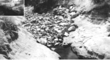
A series of riffles were installed along the brook. Plate 3 shows the lower riffle on Spencers Brook following two winter flows since construction. The riffle was constructed at the location of the head-cut shown in Plate 2. The site plan of the restoration works is shown in Figure 4. The brook is considerably straighter than the theoretical meander pattern described in Section 1.1.2. The riffle sequence was constructed to cater to the existing meanders of the brook, rather than conforming
