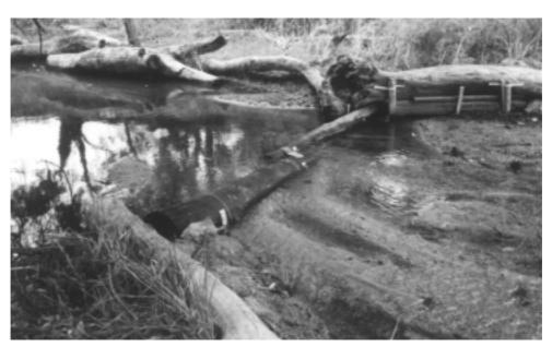
Plate 5: Large woody debris riffle built on the South Dandalup River, Pinjarra (WA).
