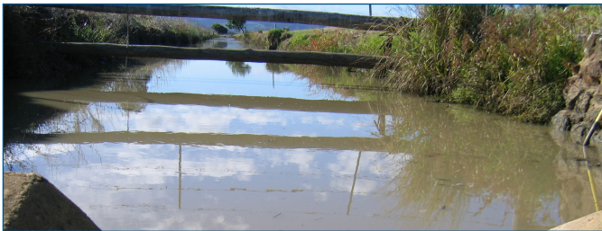
Upstream view of Samson North Drain at Somers Road – May 2006
