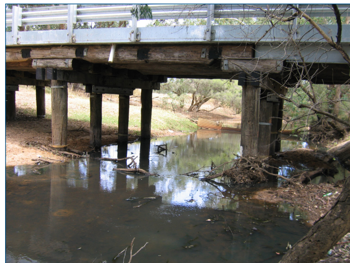
Downstream view at Patterson Road – February 2008
