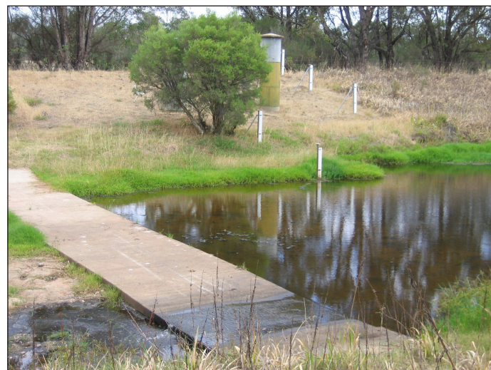
Upstream view at Dog Hill showing weir and gauging station – December 2006
