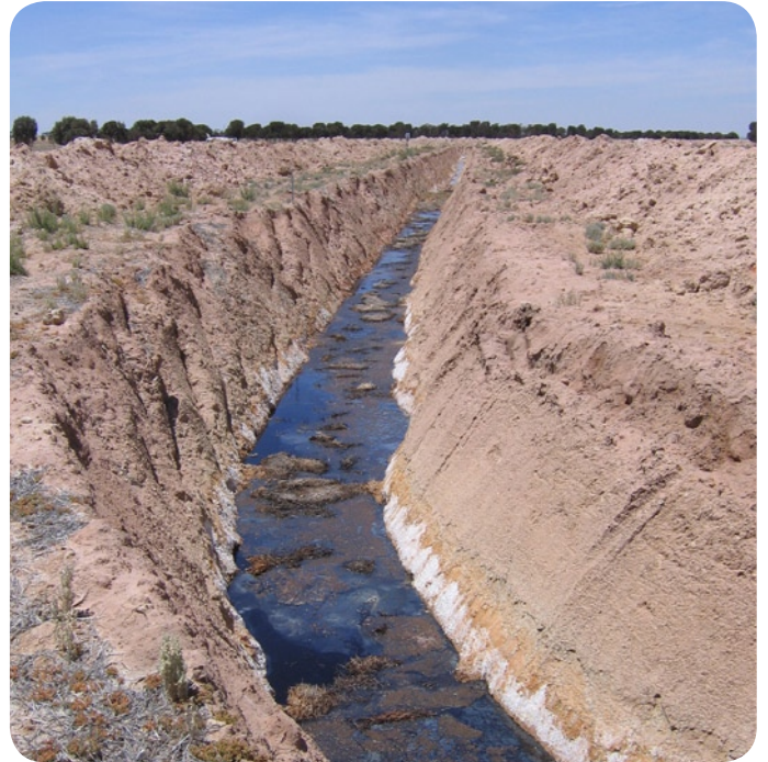
Figure 2 Example of an in-drain composting bed treating acidic drain water (in the Wallatin Creek catchment)
