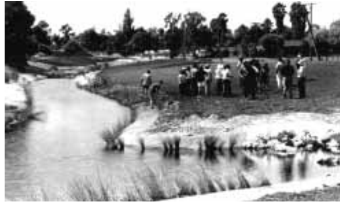
Figure 15. Channel realignment, bank stabilisation and revegetation at Bannister Creek.
