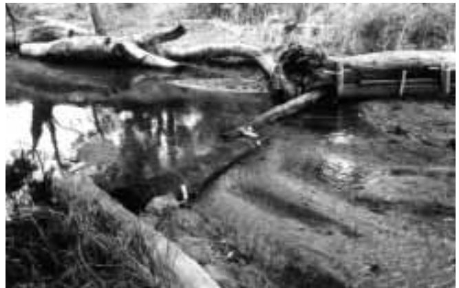
Figure 9. Log riffle and bank protection on the South Dandalup River.
