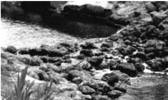
Figure 19. Riffle built on Torbay Main Drain.
