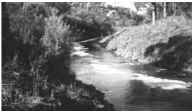
Figure 17. Revegetation along the outer bank, while access is maintained along one bank. Riffle sequence directs high flows into the centre of the channel.
