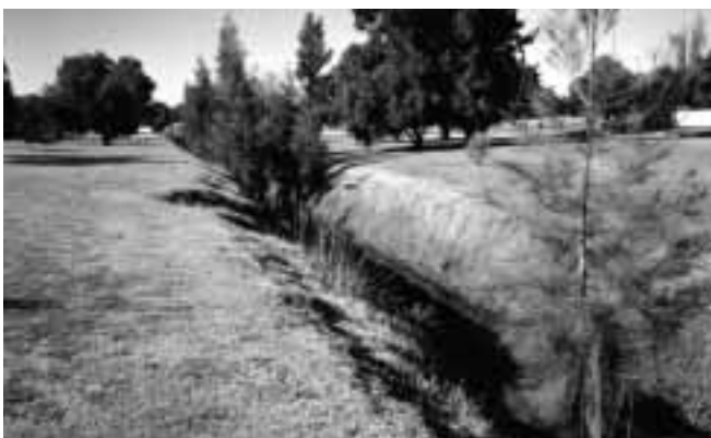
Figure 14. Bannister Creek prior to restoration works.
