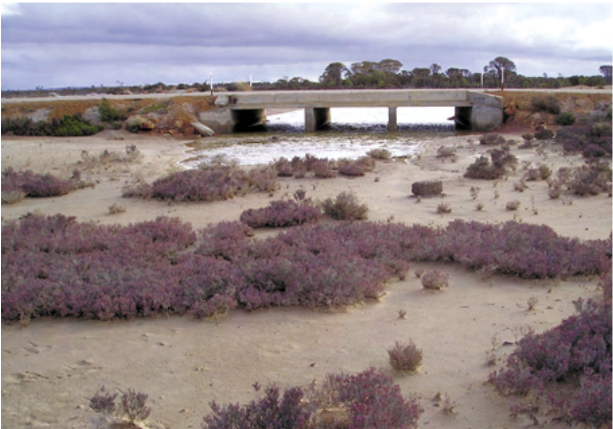
Photo 27 Box culverts on the Ardath-Yarding Road
