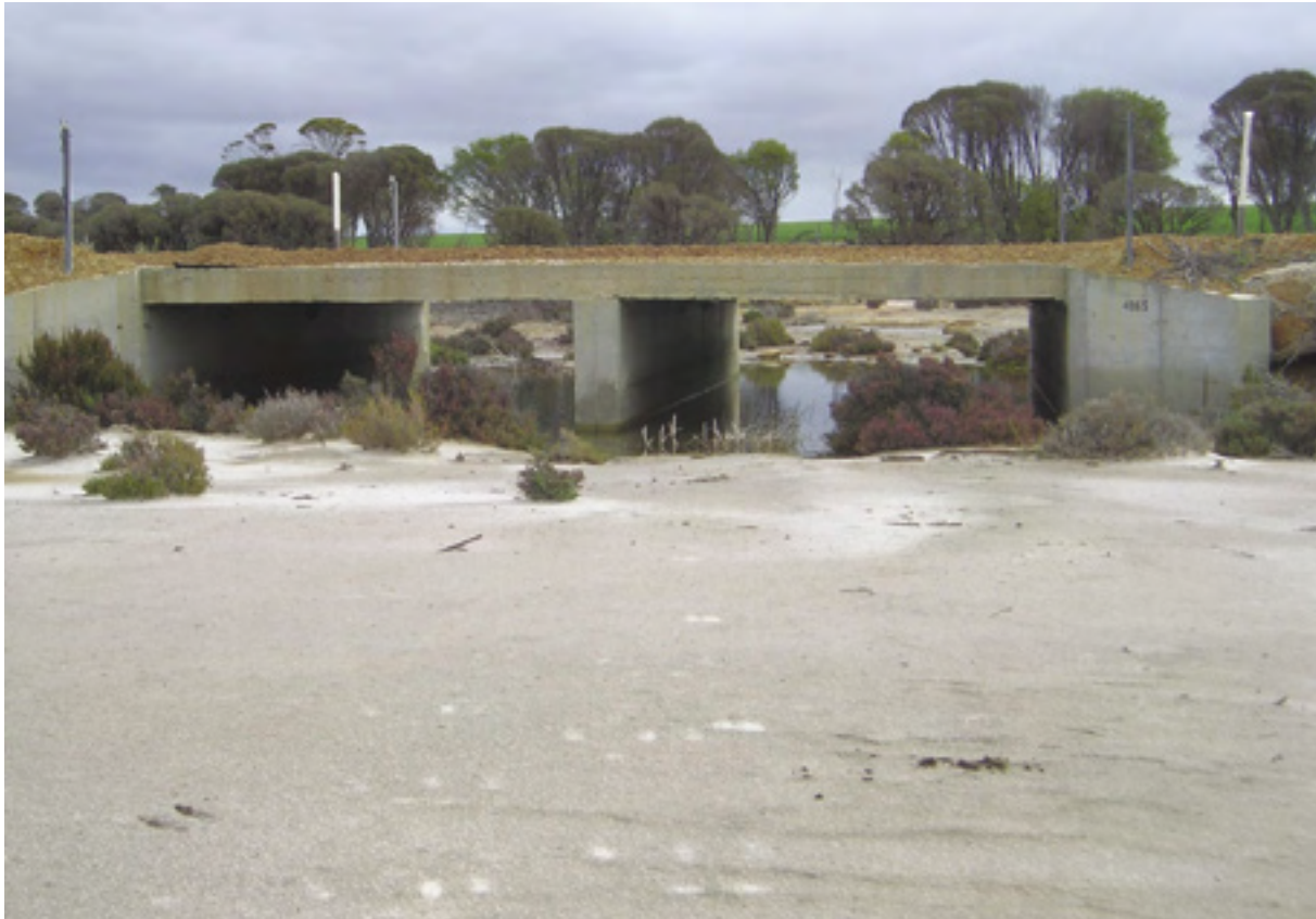
Photo 23 Box culverts on Erikin South Road
