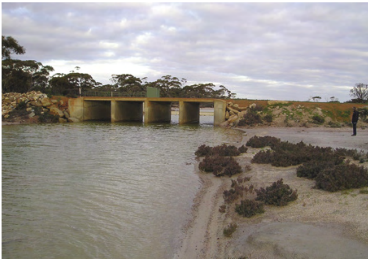
Photo 8 Box culvert structures for Kwolyin East Road
