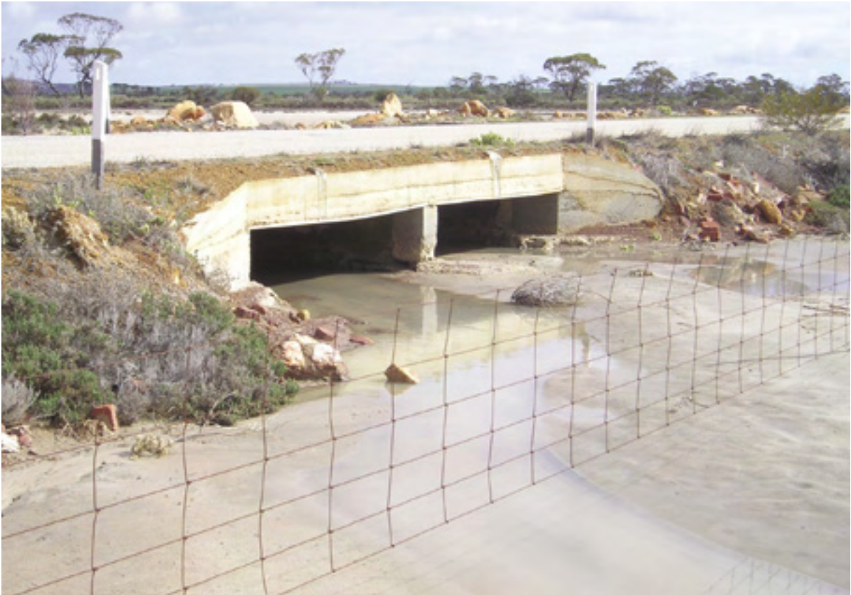
Photo 13 Box culvert on the Shackleton Road
