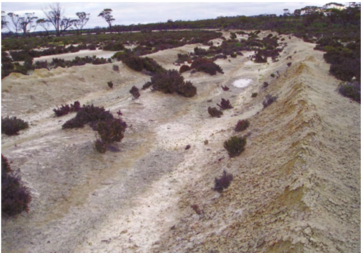
Photo 31 'W-drain' constructed for surface water management
