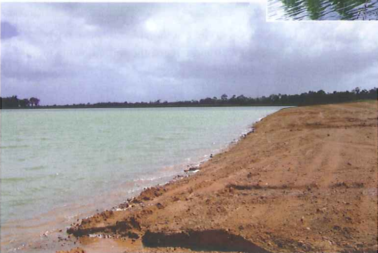
E2 grade foreshore: The banks of this dam are eroding in the absence of native fringing vegetation.
