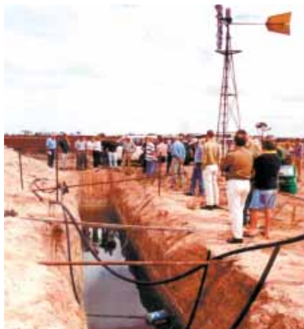
Groundwater Relief pumping, Dangin. (Photo courtesy Shane Boladeras)
