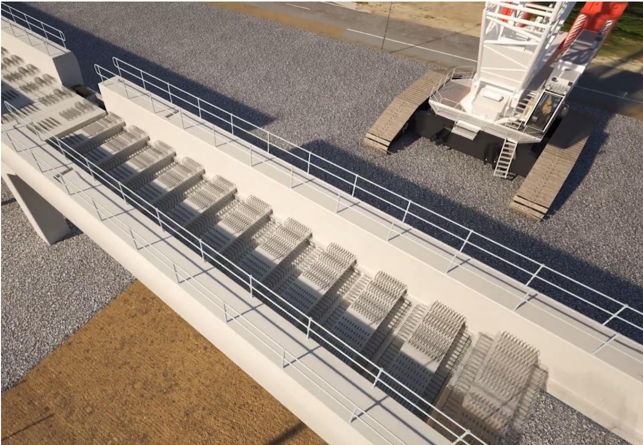
Figure 18: Bridge deck slabs being placed between the viaduct bridge beams
