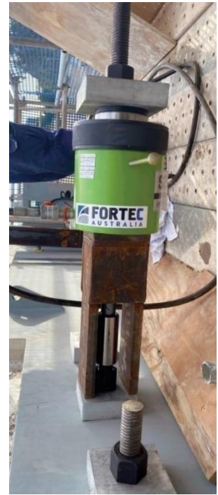
Figure 16: Example of post tension jacking
