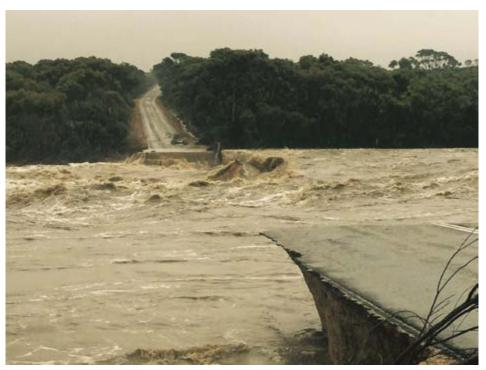
Figure 3. Flood damage to Phillips River Bridge near Ravensthorpe
