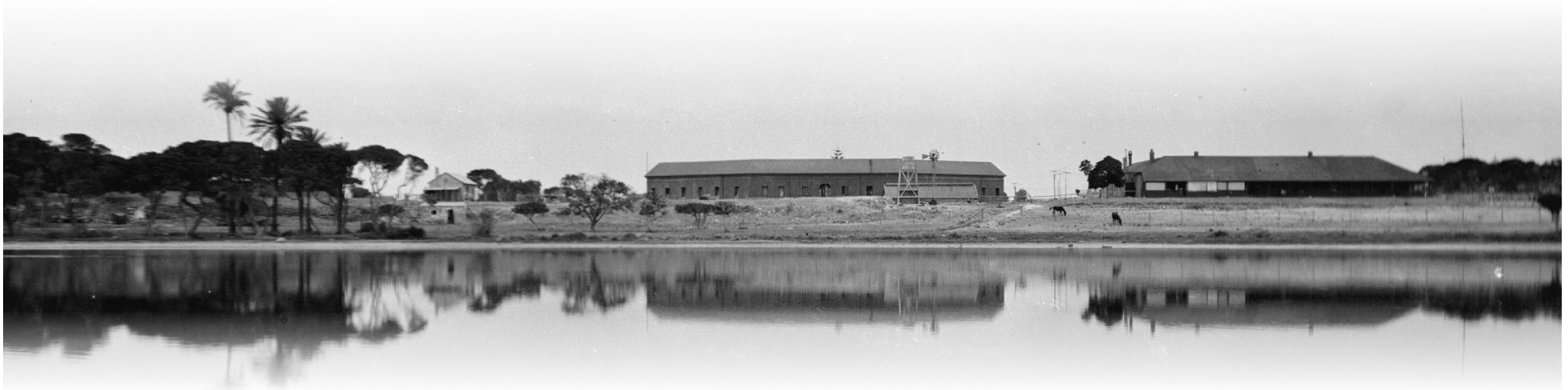
Photo credit State Library of WA
