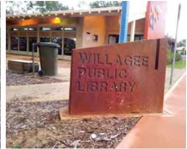
Building signage shows sign of wear and not maintained. Not clearly visible from public areas, especially at night.
