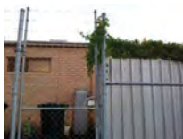
Fencing cross-bar, overgrown vegetation and lack of visibility (sheet fencing) promote a potential climbing point.
