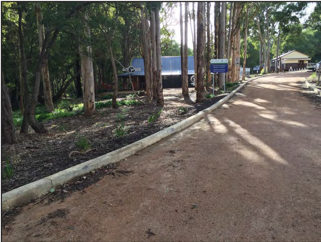
Figure 13. Example of Stabilised Gravel
